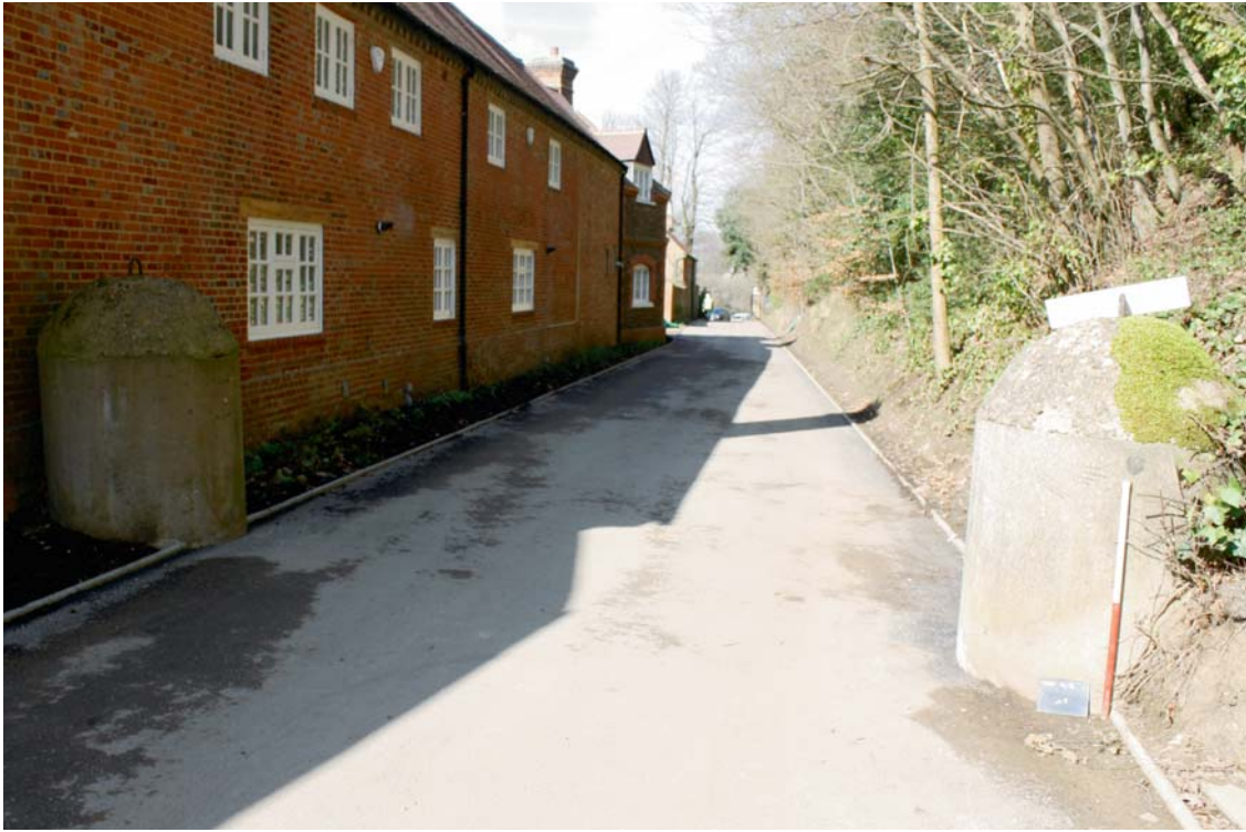
Plate 3. Anti-tank bollards, on Moor Park Drive, looking north west, Scale: 1m.
