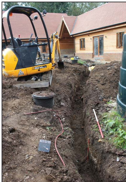
Plate 2. Trench 2, looking West, Scales: 1m and 0.50m.
